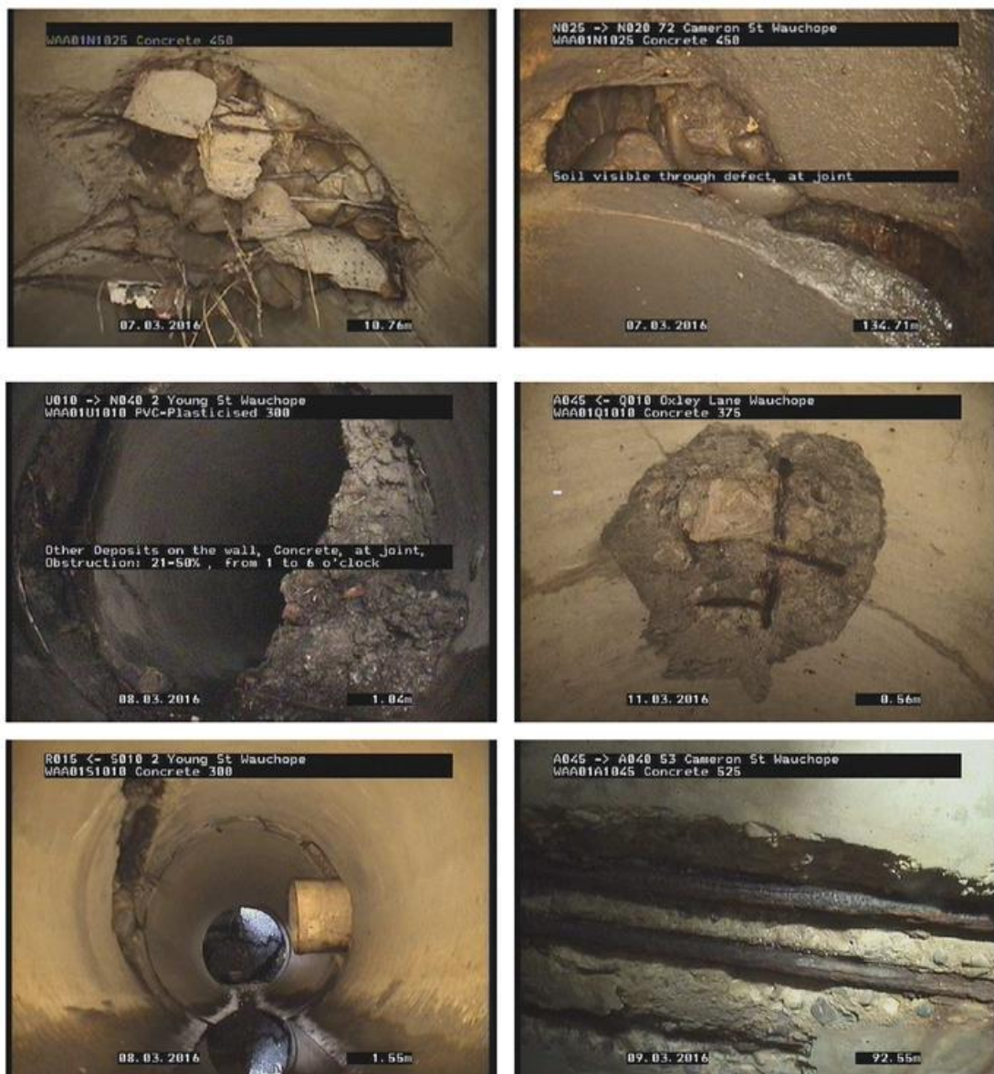
Figure 2 - Sample Images of Significant Structural Defects Within Older Piped Network
