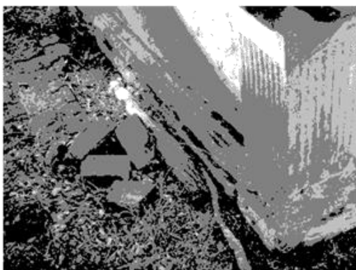
Photographs showing dislodged bricks
