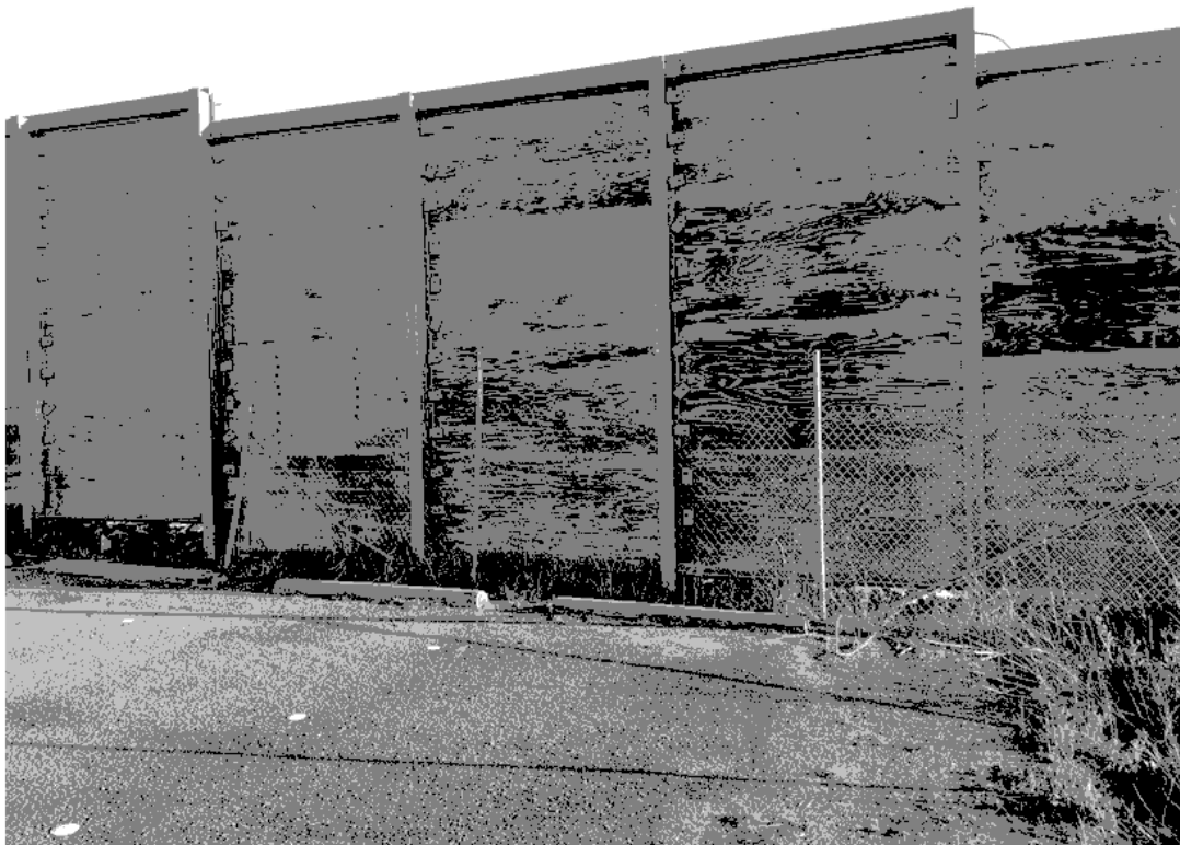
Figure 10.3 Example of a timber acoustic barrier used at the nearby I Herons Creek Timber Mill
