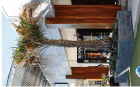
TIMBER CLAD STEEL COLUMNS
