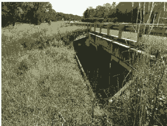
Plate 1 Three Cell Culvert System Beneath Ocean Drive
