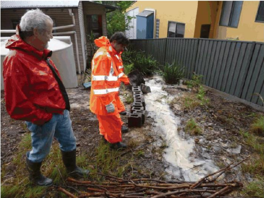
Figure 4-6 Residents unblocking culvert inlet upstream of Black Swan Terrace properties, April 2008.
