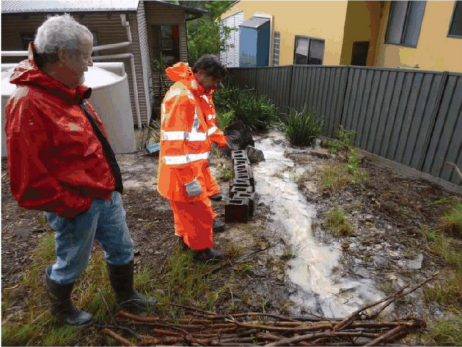
Figure 3-6 Residents unblocking culvert inlet upstream of Black Swan Terrace properties, April 2008.
