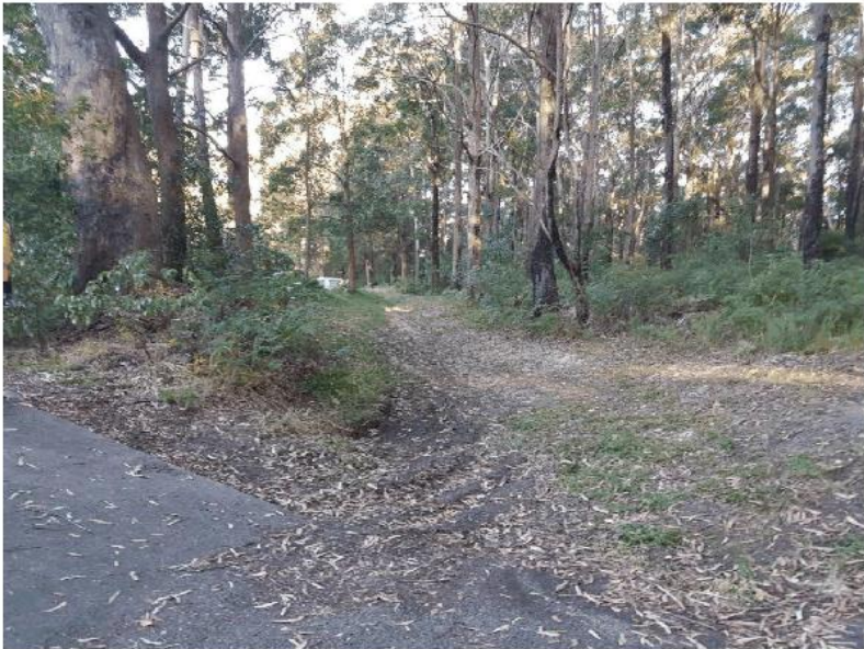
Figure 3-17 Flow diversion berm and swale upstream of development, Laurieton
