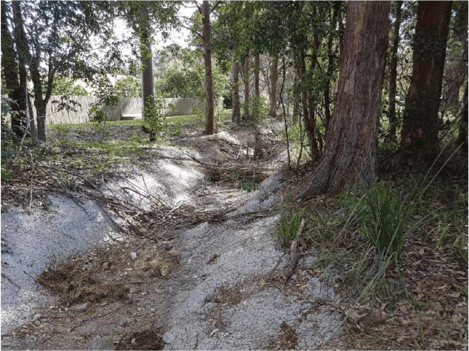
Figure 3-10 Shotcrete-lined informal channel in Lakewood
