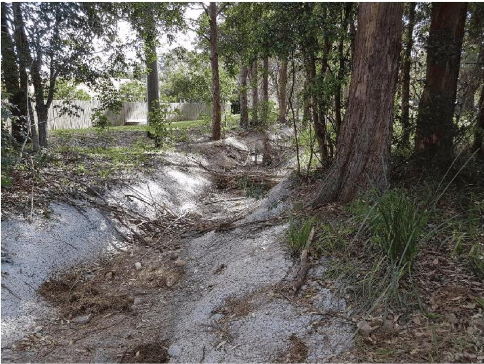
Figure 3-2 Shotcrete-lined informal channel in Lakewood
