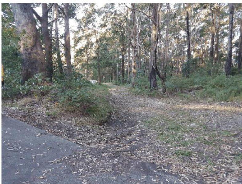
Figure 3-9 Flow diversion berm and swale upstream of development, Laurieton
