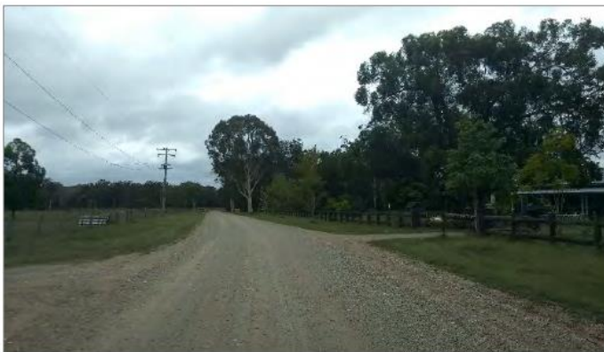
Photo 19 – View of road adjacent 170 The Hatch, Blackmans Point prior to road maintenance (photo taken 08/03/2019). Road surface recycled concrete.
