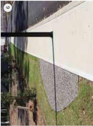
Poorly located light pole in recently completed footpath (leading to CSU student accommodation) is problematic for prams or wheelchair users
