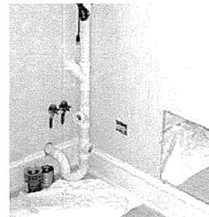
Option 2 Plumbing/Waste Line Coming through "Head Wall"
