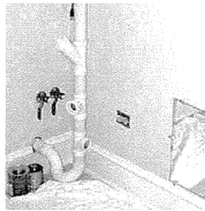
Waste Line coming Through "Head Wall"
