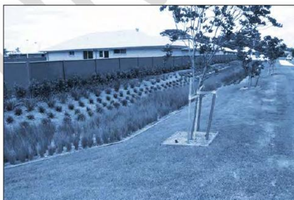
Figure 219: Constructed bioretention basin
