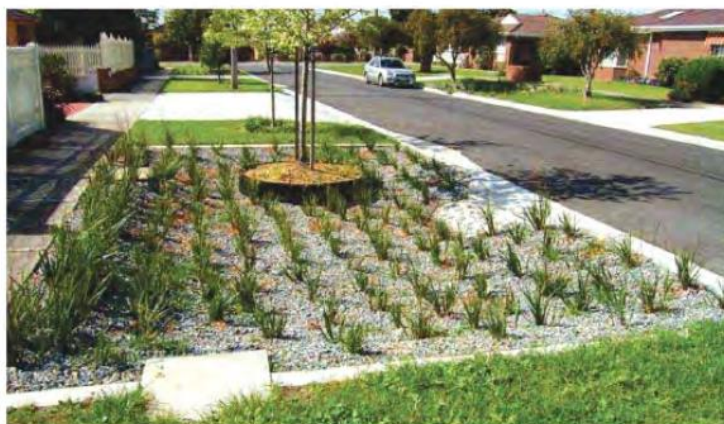
Figure 106: Example of typical bioretention system along roadway
