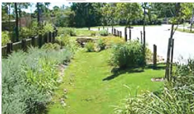
Figure 107: Example of typical grassed swale along roadway
