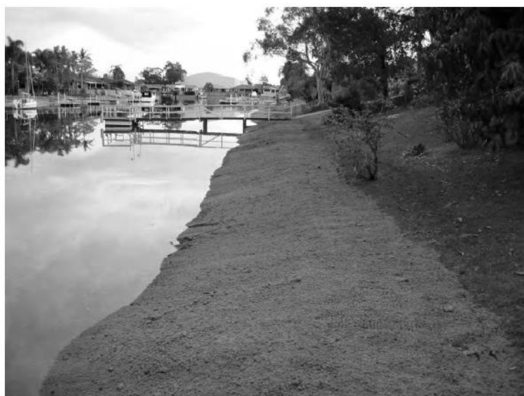
Figure 4: Restored canal beach area during 2006 maintenance dredging campaign
