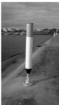
Figure 6: Flexible reflective bollards installed along crest of Broadwater Canals weir
