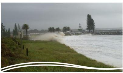
Figure 50. Town Beach showing wave overtopping rock revetment wall during lune 2016 Fast Coast Low event
