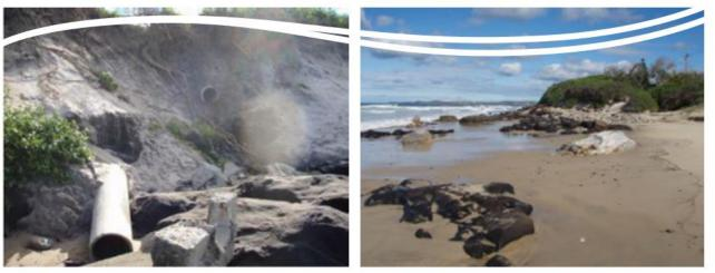
Figures 50 and 51. Coastal erosion at Lighthouse Beach causing damage to stormwater infrastructure at Jonathan Dickson Reserve.
