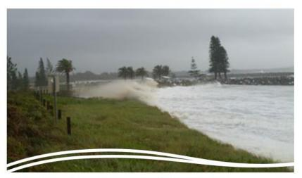
Figure 49. Town Beach showing wave overtopping rock revetment wall during June 2016 East Coast Low event.
