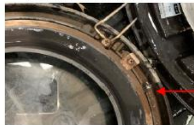
Water pooling in frame outside sealed area
