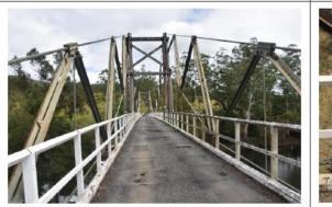
Photograph 72 – Timber Guardrails
