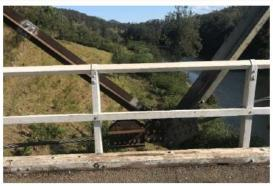
Photograph 73 – Repaired Timber Guardrails57
