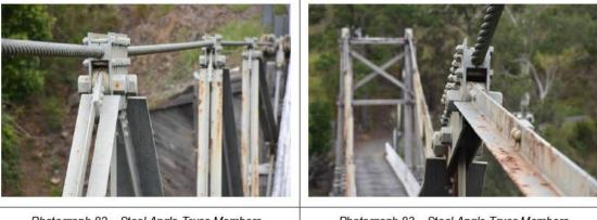
Photograph 82 - Steel Angle Truss Members
