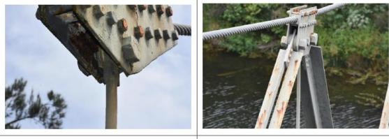
Photograph 78 - Hanging Rod Connection to Cable Truss
