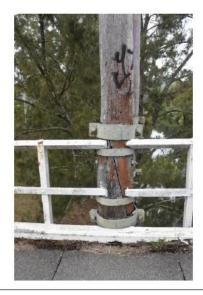
Photograph 55 – Timber Pier Scarf Joint
