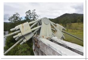
Photograph 94 - Overview of Steel Pier Bearings
