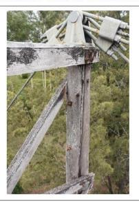
Photograph 11 – Timber Pier and Bearing
