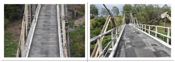
Photograph 114 – Bituminous Bridge Deck Surface
