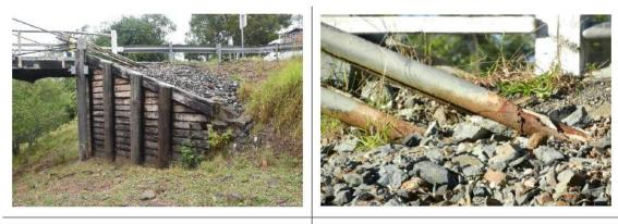
Photograph 102 - Overview of Steel Anchor Rods
