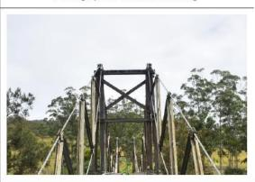
Photograph 10 - Timber Pier Bracing
