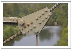
Photograph 21 – Overview of Steel Cable Node Block
