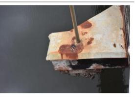
Photograph 81 - Hanging Rod Connection to Timber Cross Girder
