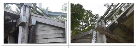
Photograph 58 – Overview of Flashed Timber Capwale
