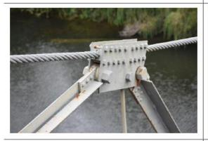
Photograph 92 – Overview of Cable Node Block
