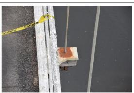
Photograph 22 - Steel Hanger / Timber Cross Girder
