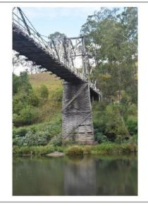
Photograph 14 - Timber Pylon & Diagonal Pier Bracing
