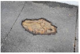
Photograph 117 – Deteriorated Plywood and Bituminous Bridge Deck Surface
