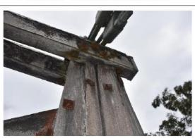
Photograph 9 – Timber Pier Head and Brace
