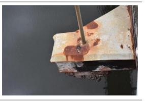
Photograph 65 – Typical Timber Cross Girder to Hanger Connection
