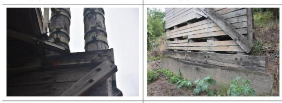
Photograph 56 - Timber Piers Strapped with Steel Bands
