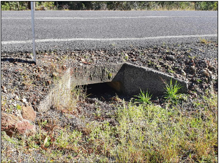
PHOTO 1 EAST END OF CULVERT - TO BE EXTENDED
