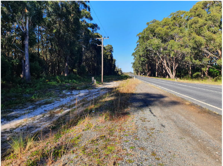
PHOTO 4 OPPOSITE DRIVEWAY LOOKING SOUTH
