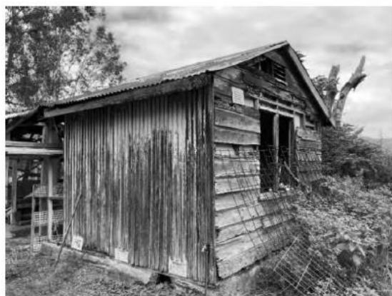
Old shed that had partially collapsed. Wall on western side was of corrugated fibre cement construction.
