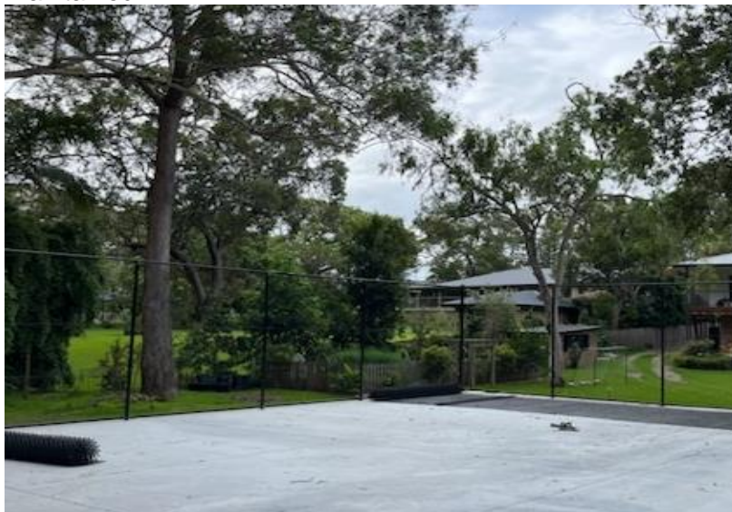
Looking North West from tennis court
