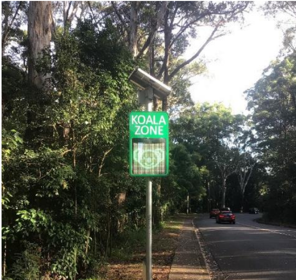
Image 3 - Typical vehicle Activated Sign - Lord Street, Laurieton
