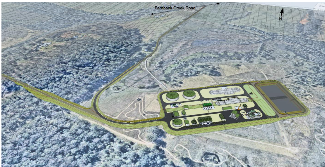
Figure 1: The proposed Thrumster Wastewater Treatment Plant concept design 3D model. The critical elements of the plant are located on the southern section, which has been raised to the FPL4, being just above the PMF level. The northern section has been raised to FPL3.
