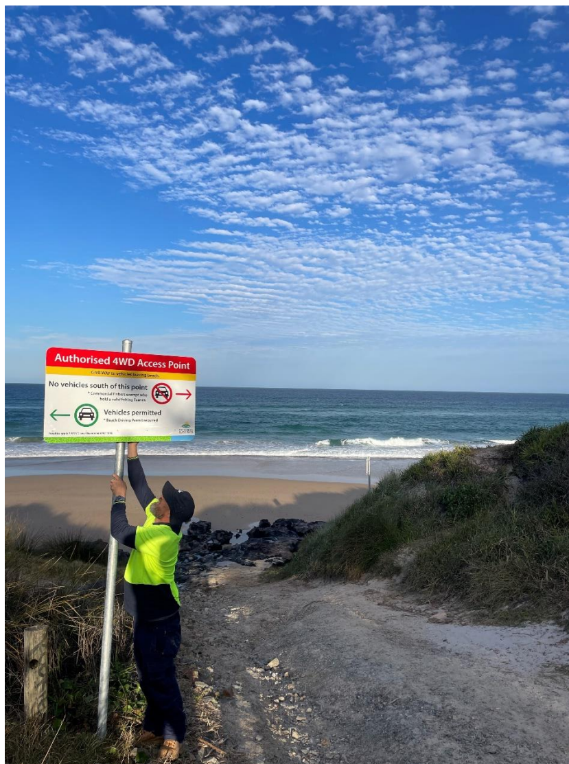
Figure1: Installation of Sign at Beach Access Point at Lake Cathie
