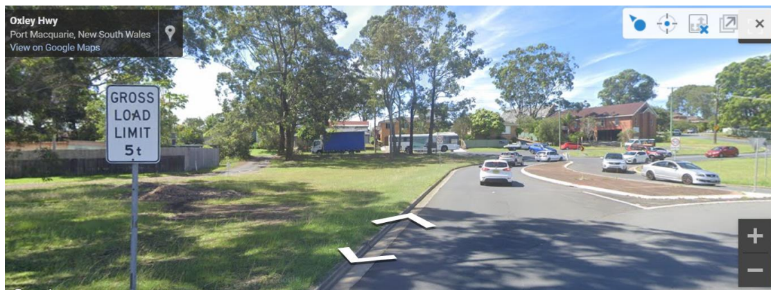
Image 2 - southern entry to Clifton Drive (Google Streetview 2024)
