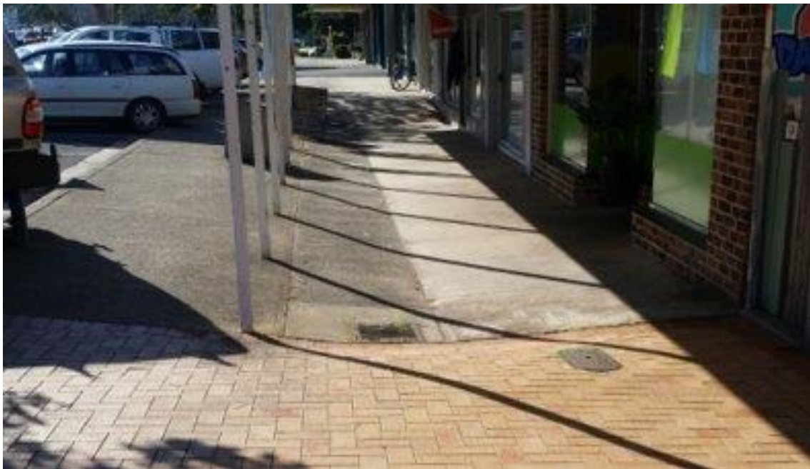
Figure 5 - Steep eastern side of crossing Option 2 to be addressed.
