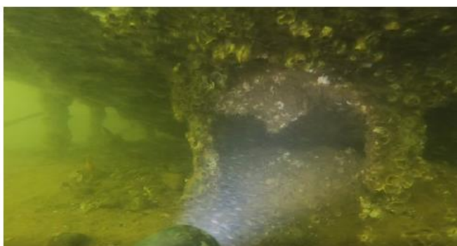
Figure 5: Section loss Pier 3 Pile 2.
