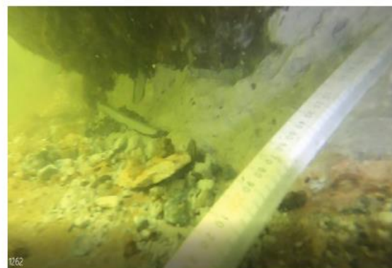
Figure 4: Section loss Pier 3 Pile 1.
