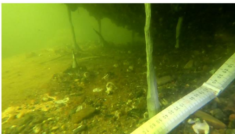
Figure 1: Still photo from video captured during underwater inspections of Pier 4, Pile 2 showing approximately 88% erosion of a section of the foundation pile.
